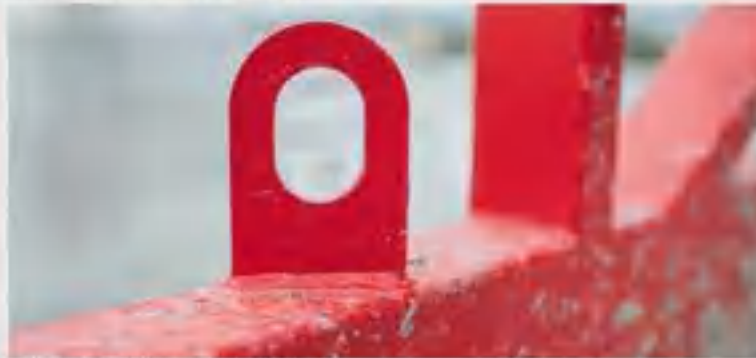
Fixing of the crane's sling.
