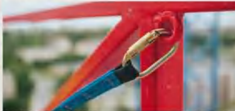
anchoring points for PPE
